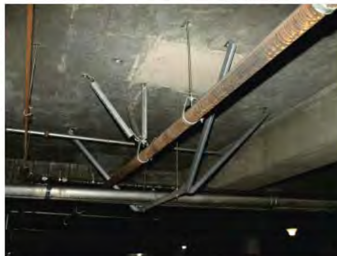
Figure 6.4.3.1-7 Transverse bracing with J-hanger and strut at the restraining bolt. Note that longitudinal brace shown is ineffective because the J-hanger can slip along the length of the pipe; a pipe clamp or equivalent is required for a longitudinal brace (Photo courtesy of Cynthia Perry, BFP Engineers).
