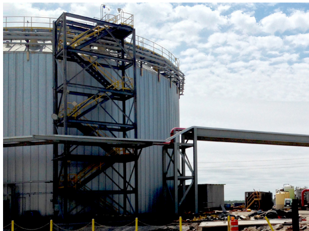
Figure 1. Molten sulfur tank with required insulation provides uniform flow to the forming unit.
